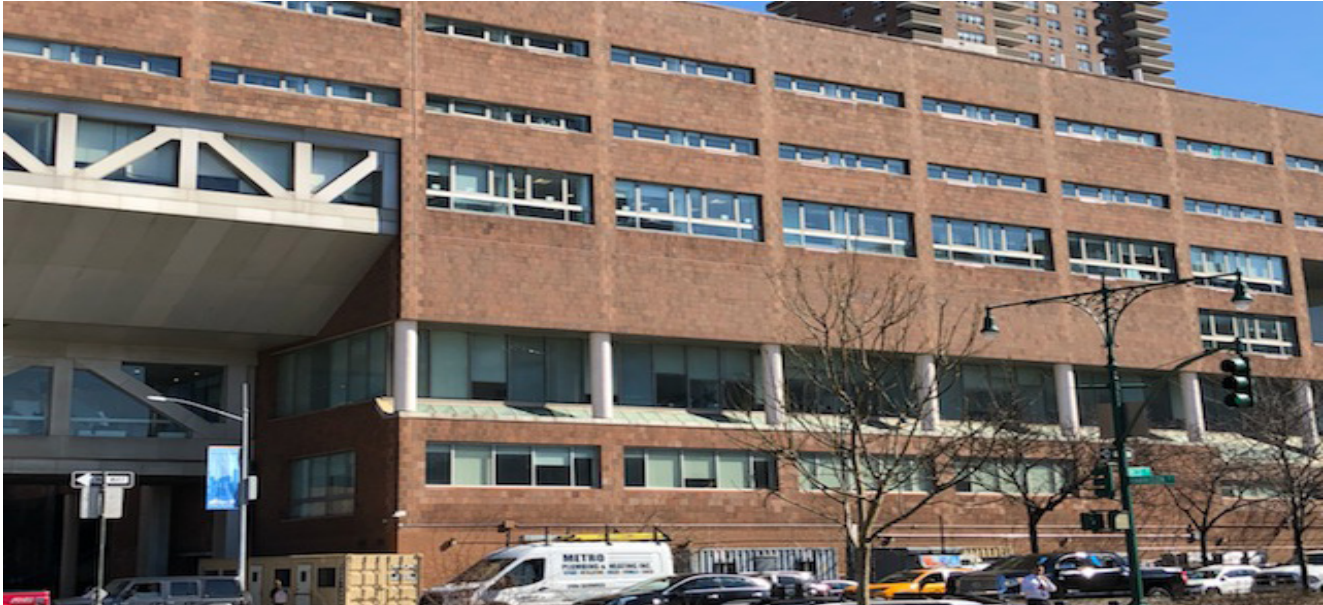
Borough of Manhattan Community College, $5.9 million façade restoration.
