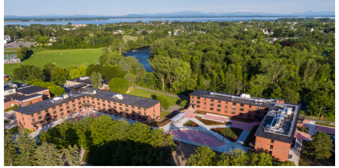
SUNY Plattsburgh Kent & Maccomb Halls received $17 million in renovation/upgrades.
