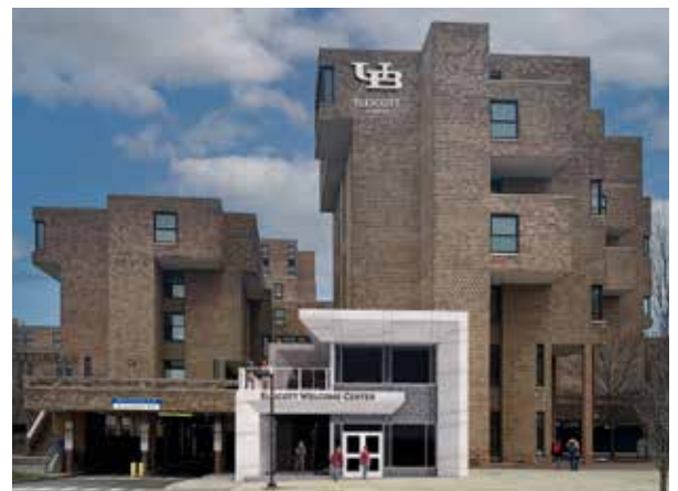
University at Buffalo Ellicott Complex entrance renovation
