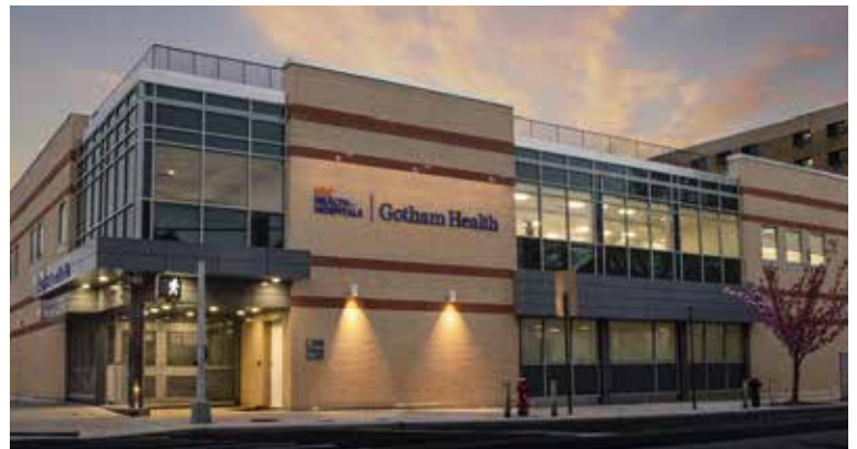
LEED Silver NYCHH/Gotham Health Vanderbilt
