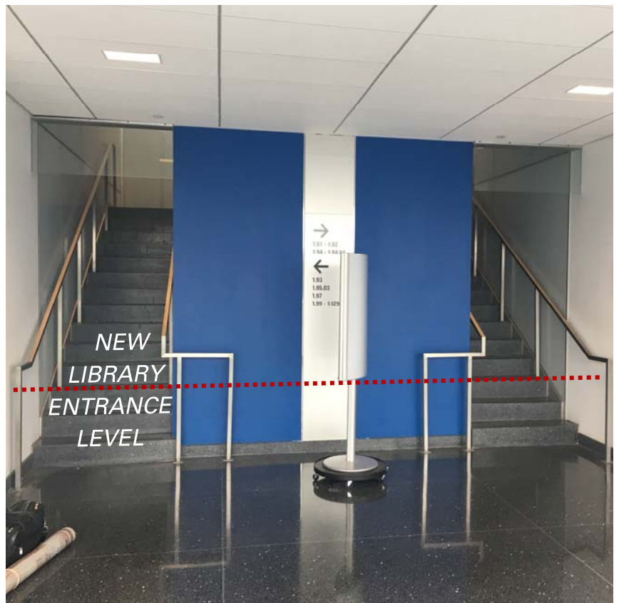
View of the location of the new library entrance onto the John Jay Commons.
