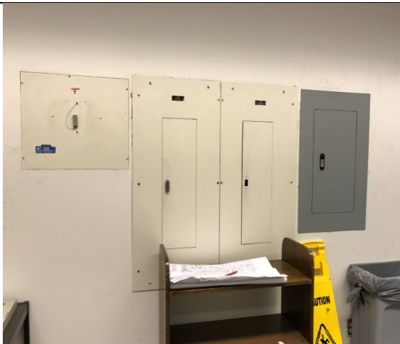
Photo E3-Existing Panelboards to be Replaced
