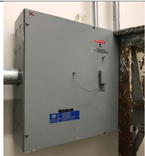
Photo E4- Existing Lighting Control Panel 'LVR'
